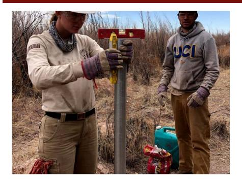
(Left) Prior to setting the brace with concrete corps members checked to ensure that the brace was standing straight.
