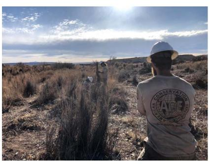
(Left) Corps members line out and set t-posts that will help support the wire. The process here is referred to as "Shooting the Line." One person stands at the brace and directs those working with them where to place the post.
