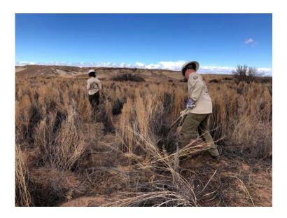
(Left) Prior to constructing the fence line corps members had to remove invasive camelthorn and grasses so that wire could be run without obstruction.
