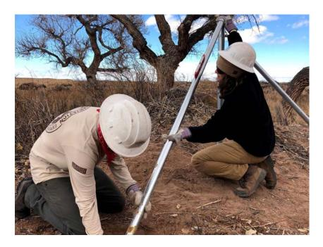
(Left) Setting the supporting angle posts for corner braces.
