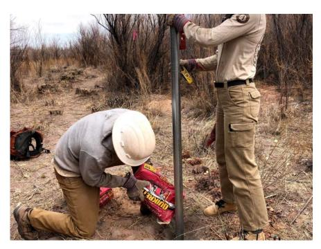
(Left) Concrete being poured into the post hole prior to adding water to set the post.
